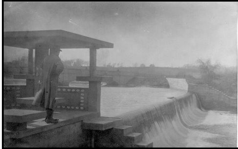
Island Woolen Mills Dam observation deck and spillway circa 1910. Photograph courtesy Sauk County Historical Society Trimpey Collection.
