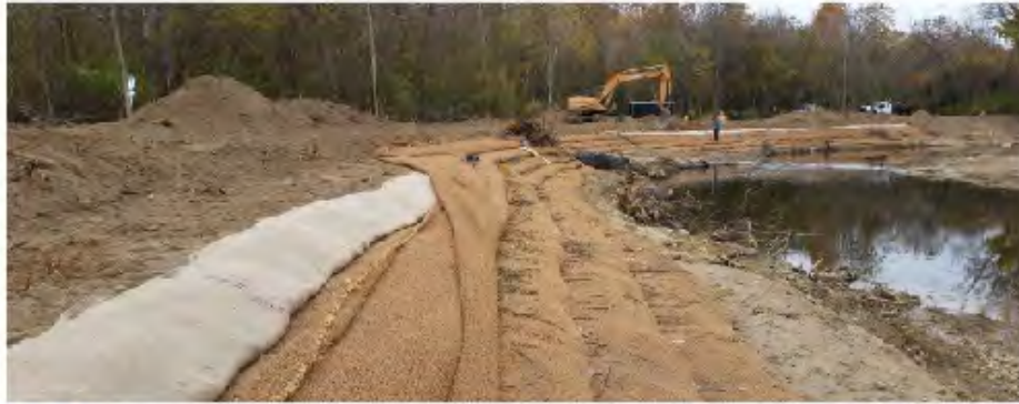
FIGURE 7: Vegetated geolifts designed and installed (Oct 31, 2015) on Eagle Creek by FLR
